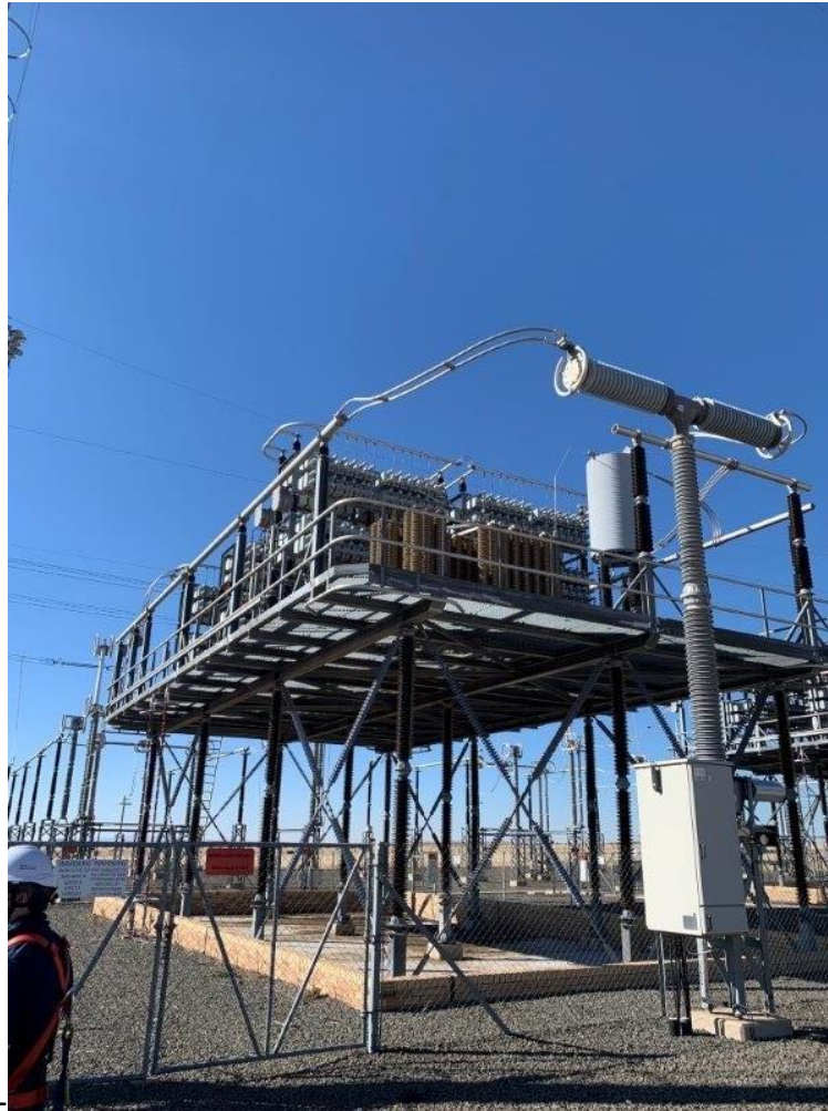
Figure 1: 400kV, 292 MVar Serumula Series Capacitor No. 1 Blue phase
